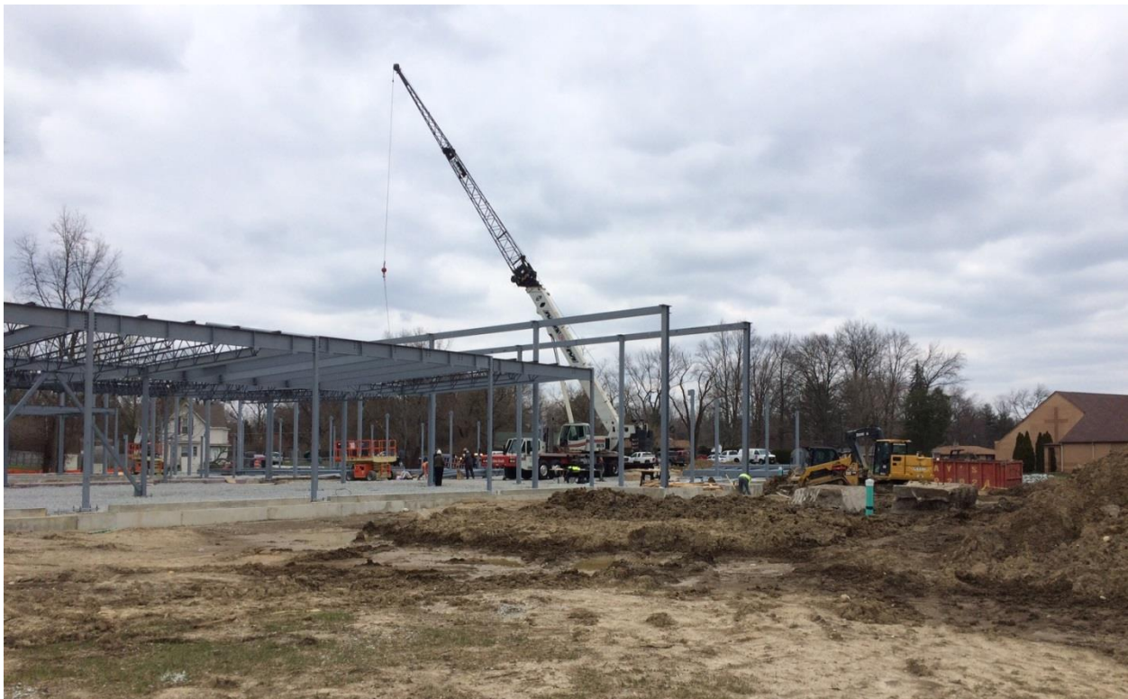
Project Site on April 10, 2018 View from the southwest showing the installation of steel columns, beams and roof joists.
