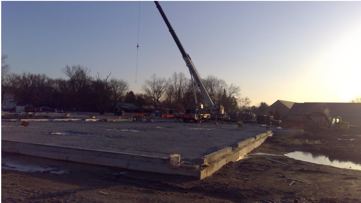
Project Site on April 5, 2018 with the completed stone base for the concrete slab and the placement of the crane.
