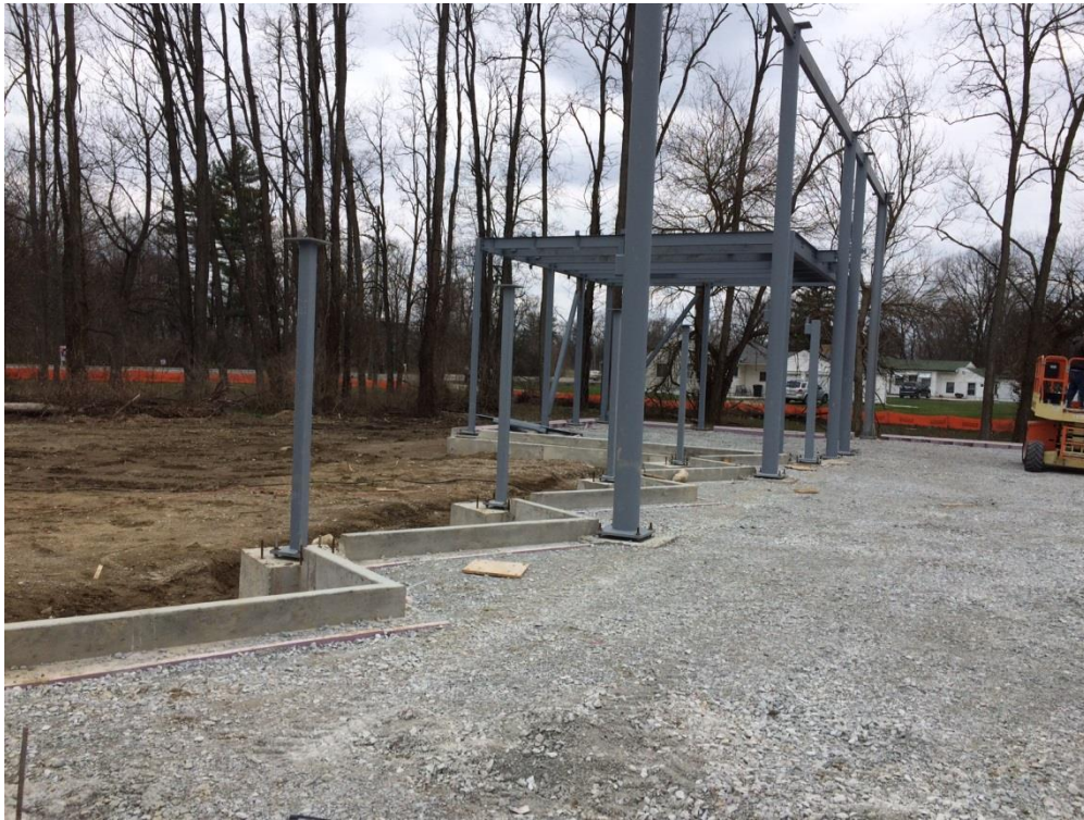
Project Site on April 10, 2018 View looking northwest of the saw-tooth seating area.
